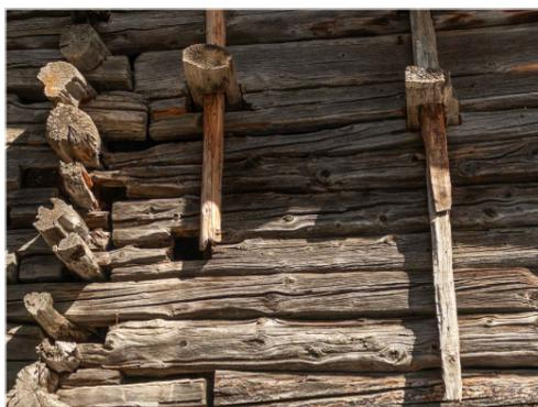
Fig. 36 Log wall structural tying and reinforcement. Nicolau Vilaró
